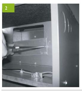
**STEP 3.** Slide the kit into the duct and fasten the element (e.g. attachment and wires).
