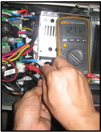
10.4.5 Open circuit or short circuit of temperature sensor diagnosis and solution(E5/E6)
