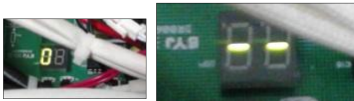
PIC3 :Main board LED when power on and unit standby.
