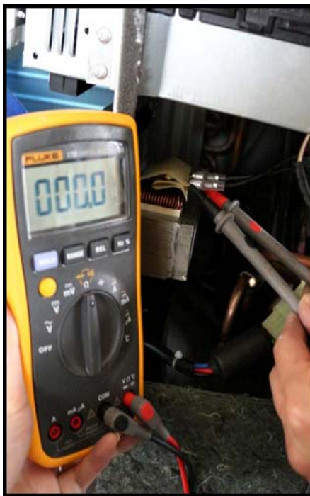
Fig. 33 — Test the Reactor Resistance
