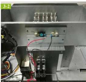
**STEP 4.** Install the circuit breaker into the mounting rail. Knock off the reserved cover for breaker in blower access panel prior to put it back to the unit.
